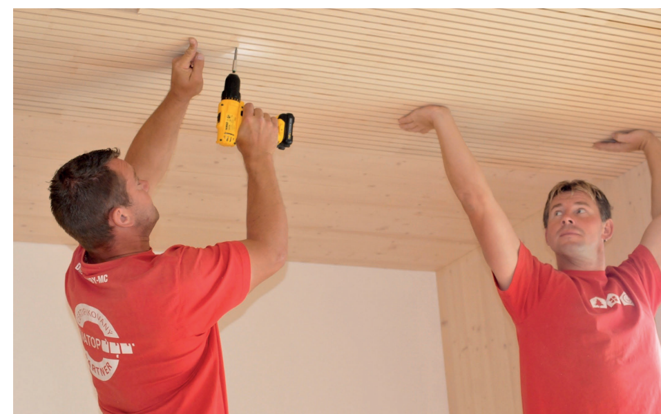
INSTALLATION OF THE NOVATOP ACOUSTIC CEILING BY MC FRAMES TEAM (COOPERATION OF EUROPEAN AND SOUTH AFRICAN BUILDES)
